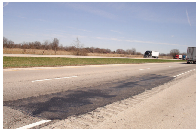
Figure 5.1 Rehabilitation of the SPS9-A study site.
